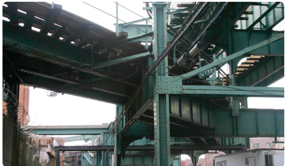
Figure 24: Broadway Junction elevated structures
