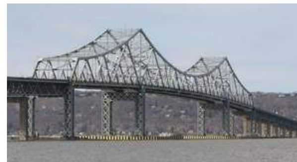
The Tappan Zee Bridge is pictured from Tarrytown March 22. (Mark Vergari/The Journal News)
