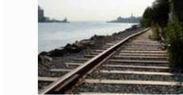
Michael McWeenyTHE PROBLEM: The North Shore rail right-of-way is available, but the tracks have fallen into disrepair. Cost to rebuild: $400 million.
